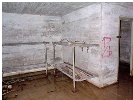
Photographs above show some of what is behind the locked steel doors of the gun emplacements on Tomaree Headland
