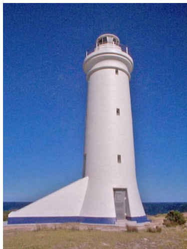
Point Stephens Lighthouse, now automatic and solar powered
