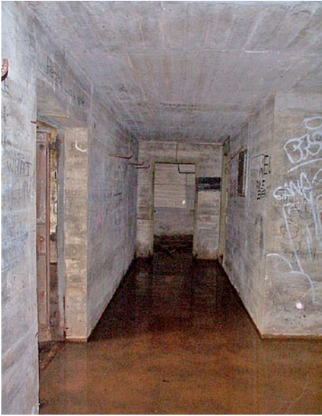
Behind the locked steel doors of the gun emplacements on Tomaree Headland
